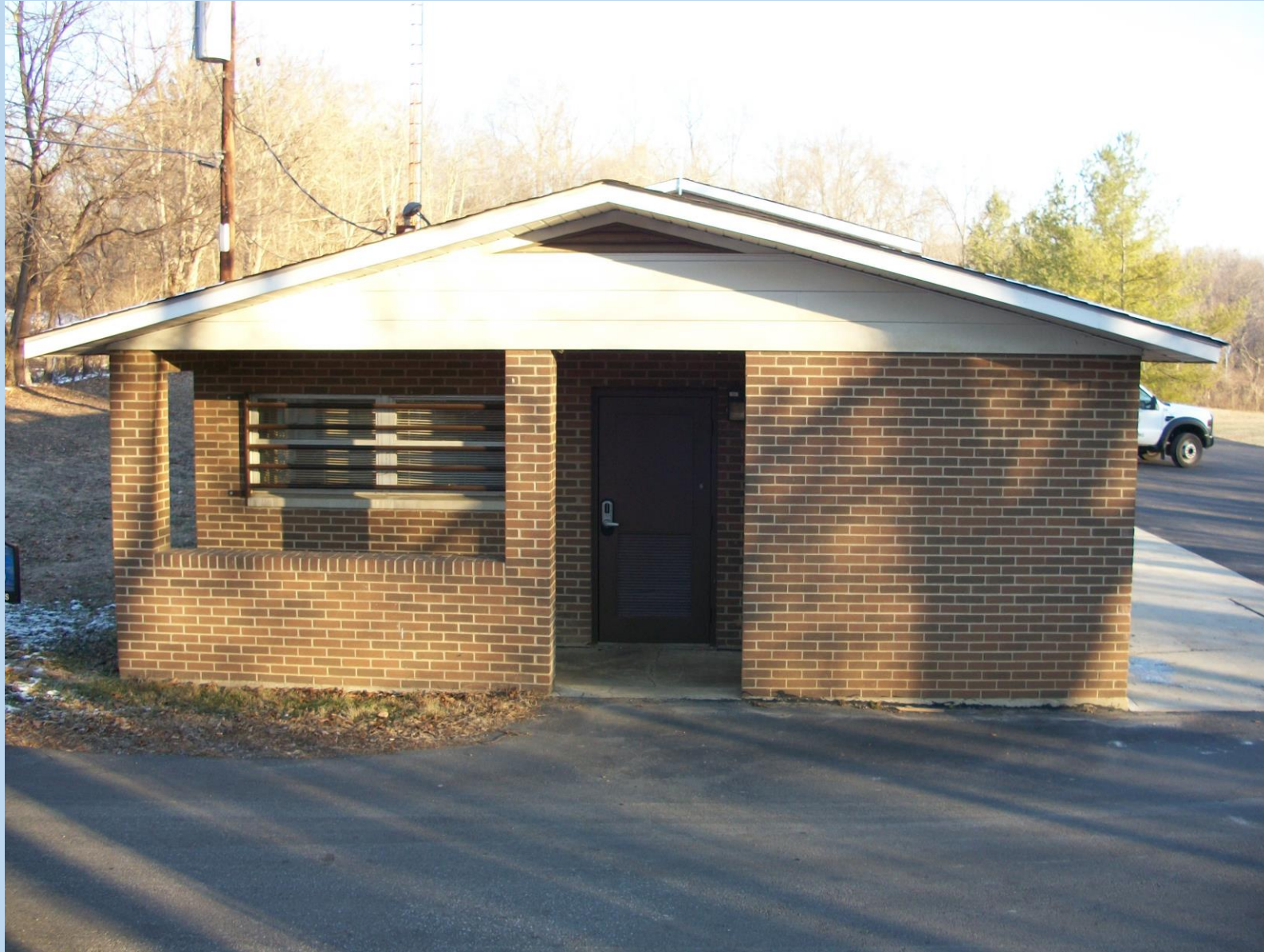
City of Loveland Water Treatment Plant
